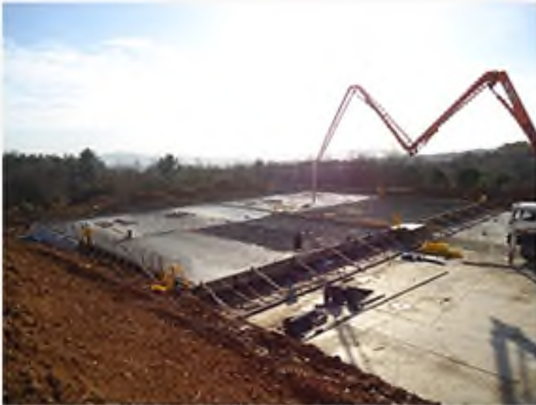
ASIAN REGION MISCELLANEOUS DRINKING WATER CONSTRUCTION – 10
