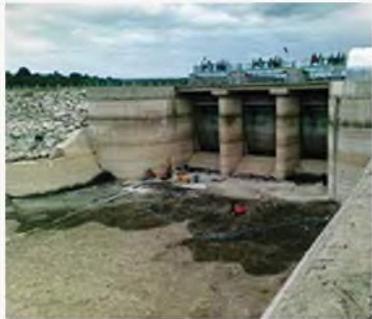
PABUÇDERE DAM INJECTION AND REINFORCEMENT WORKS
