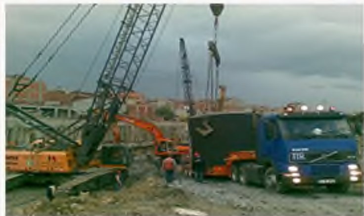
PIPE INSTALLATION WORKS WITHIN THE SCOPE OF FIRUZKÖY WASTEWATER TUNNEL
