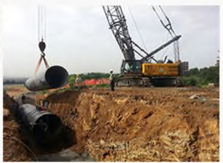
ASIA REGION REINFORCED CONCRETE PIPE REHABILITATION CONSTRUCTION 2
